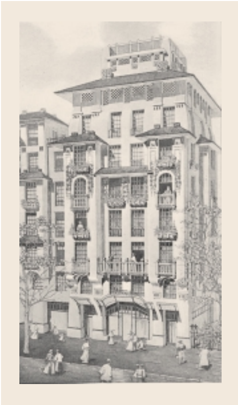
A Fondation apartment block, Augustin Rey
