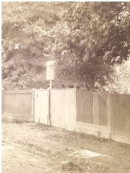
'A part of Baron Rothschild's property at Acton which fronts the Uxbridge Road showing the strip of land next to the palings under which the wires of The Electric Telegraph Company are fixed' (BL8735.dd.10: photo 'C')
