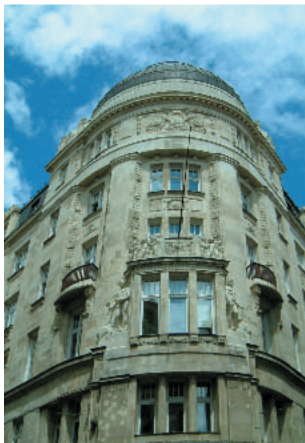
Nádor utca 14, Budapest, the headquarters of the Hungarian General Credit Bank from 1913 is today occupied by the Hungarian Ministry of Finance. Photograph by Miljenko Marohnić.
