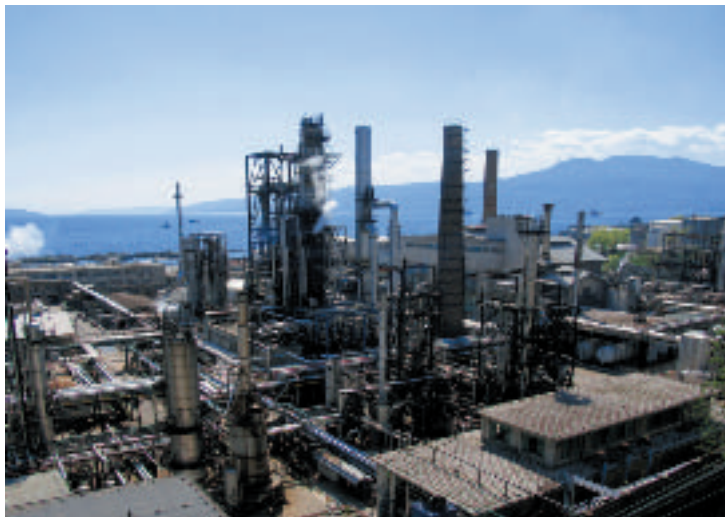
The refinery today, with an annual refining capacity of 4.5 million tons of crude oil. Photograph by Zoran Žimirić.
