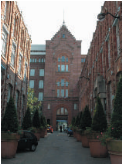
Main entrance to the CAMT, Roubaix, the former Motte-Bossut cotton mill.
